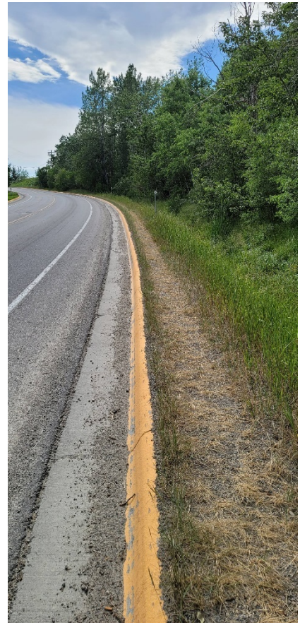
Figure 2 Lack of connectivity on Brewery Hill
