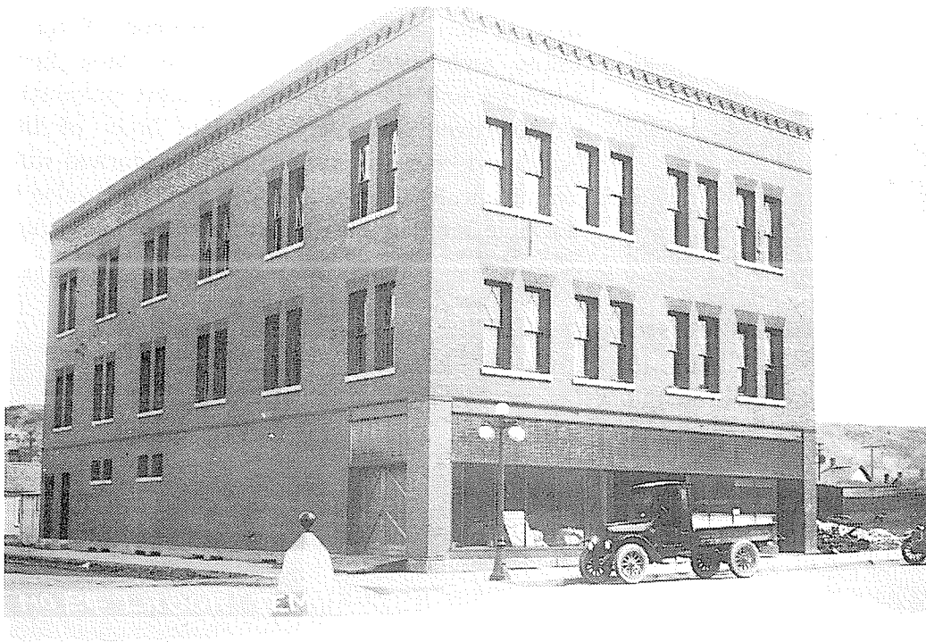
Fig. 5. Excellent example of a 1920s-1930s metal mullion and leaded glass transom storefront.
