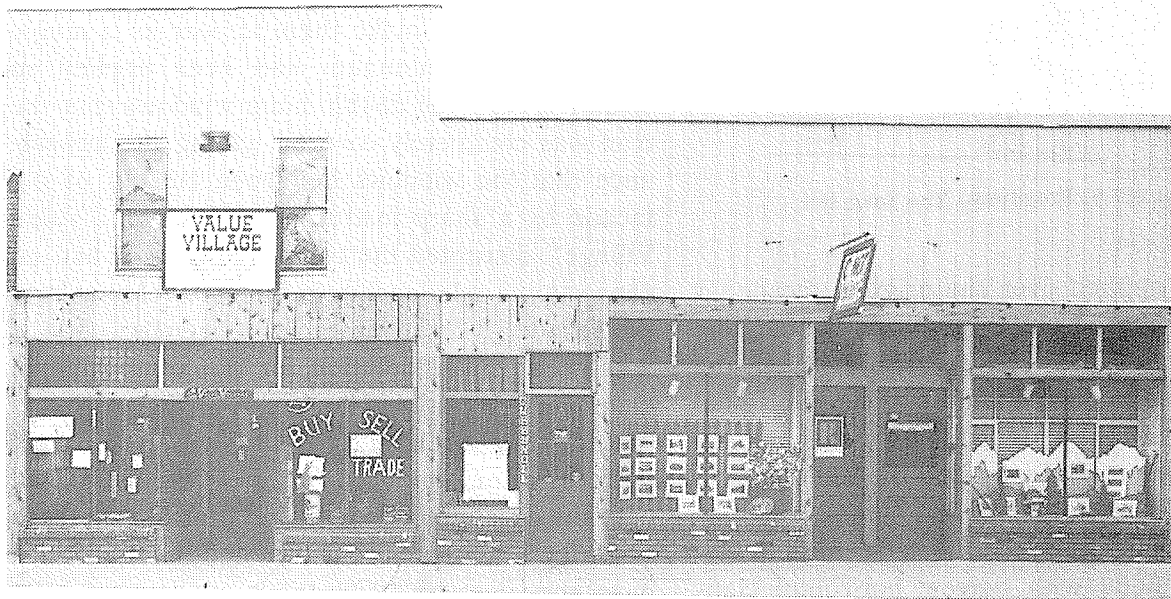
Fig. 61. 108, 108½, 110 S. Broadway before rehabilitation
