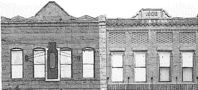
Fig. 7. Name and date stones above cornice add interest and sense of past to building.
