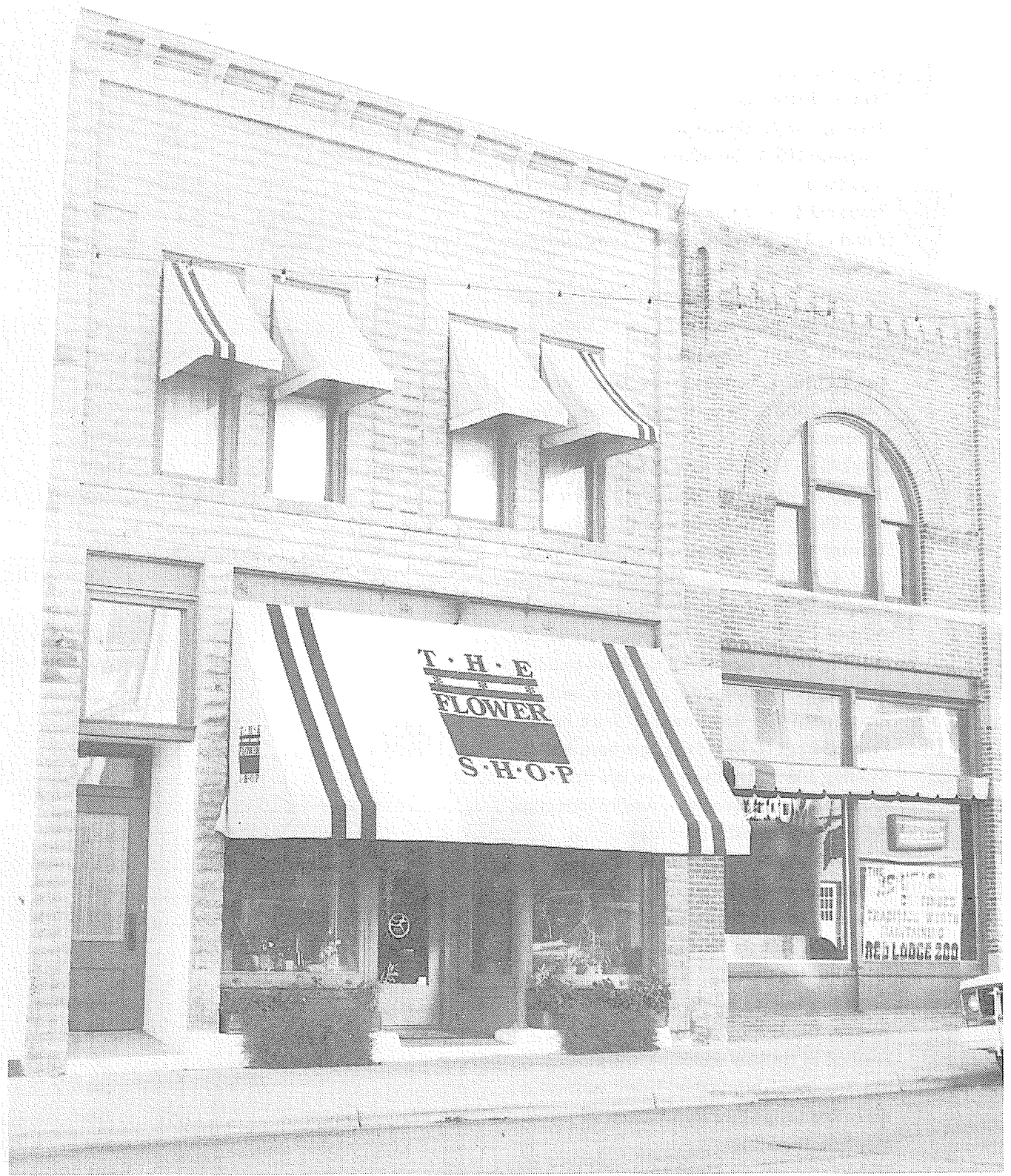
Fig. 1. Recently rehabilitated storefront, 26 N. Broadway.
