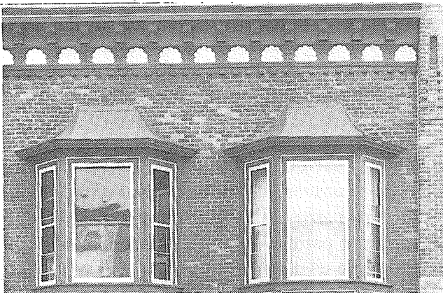
Fig. 8. Original sheet metal cornice imitates sculpted stone ornament.
