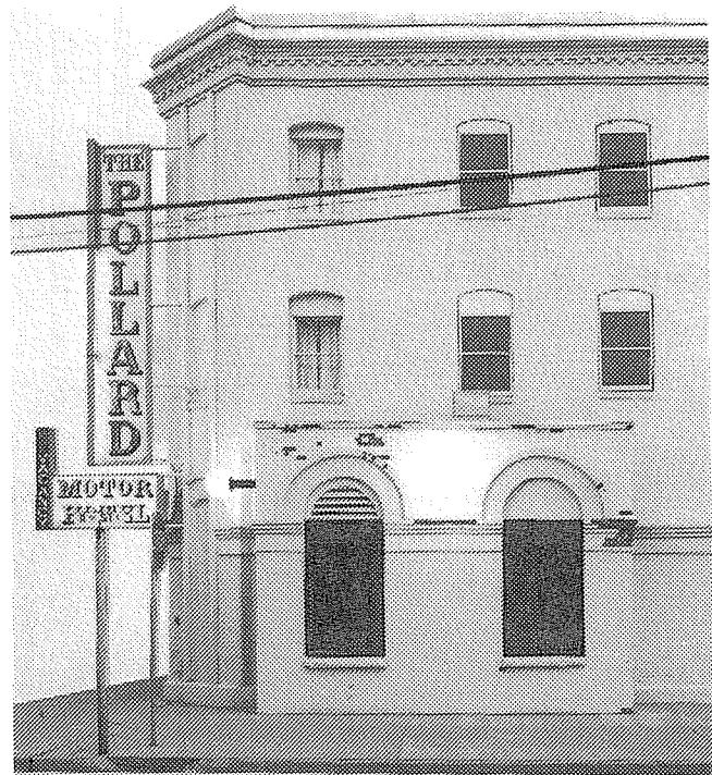
Fig. 54. 11th Street side of Pollard showing existing sign.
