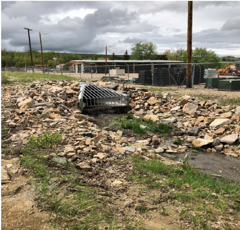
View of MDT outfall looking northwest.
