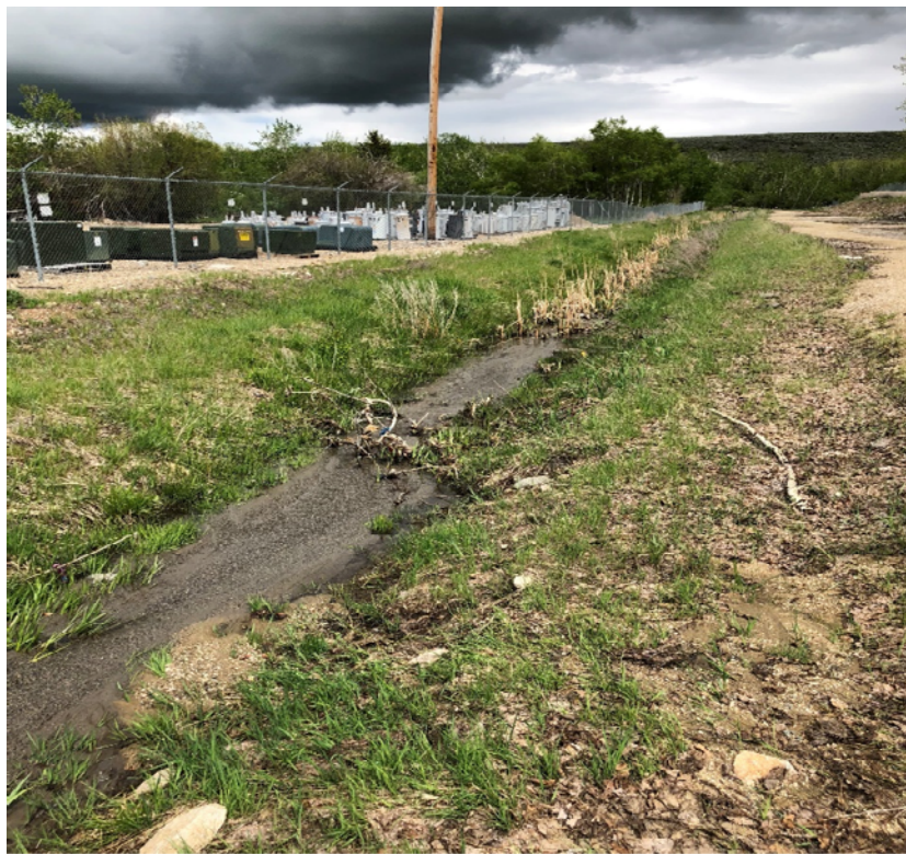
View of MDT outfall ditch looking east toward Rock Creek.
