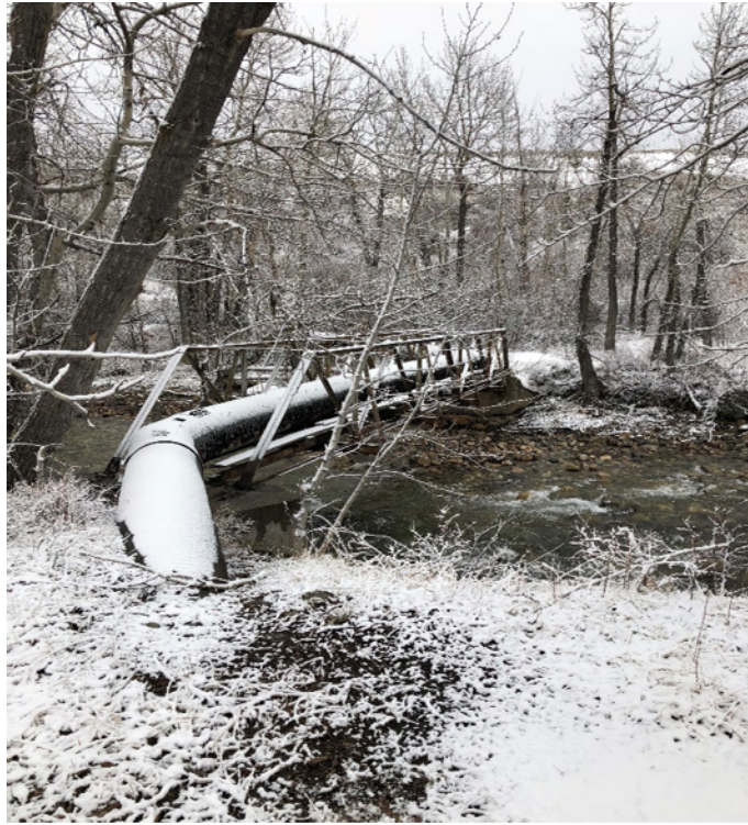
View of abandoned sanitary sewer aerial crossing of Rock Creek, looking north east.
