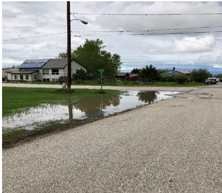
Localized flooding at the intersection of 6 th Street and Cooper Ave.
