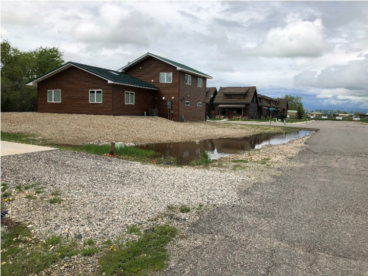
Figure 14: View of intersection of 2 nd St. and Cooper Ave. Looking north
