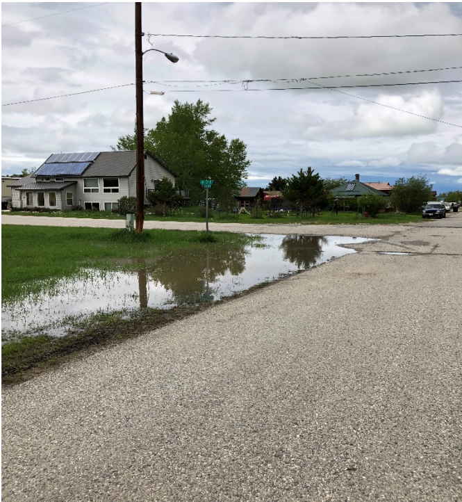
Figure 13: View of intersection of 6 th St. and Cooper Ave. Looking north
