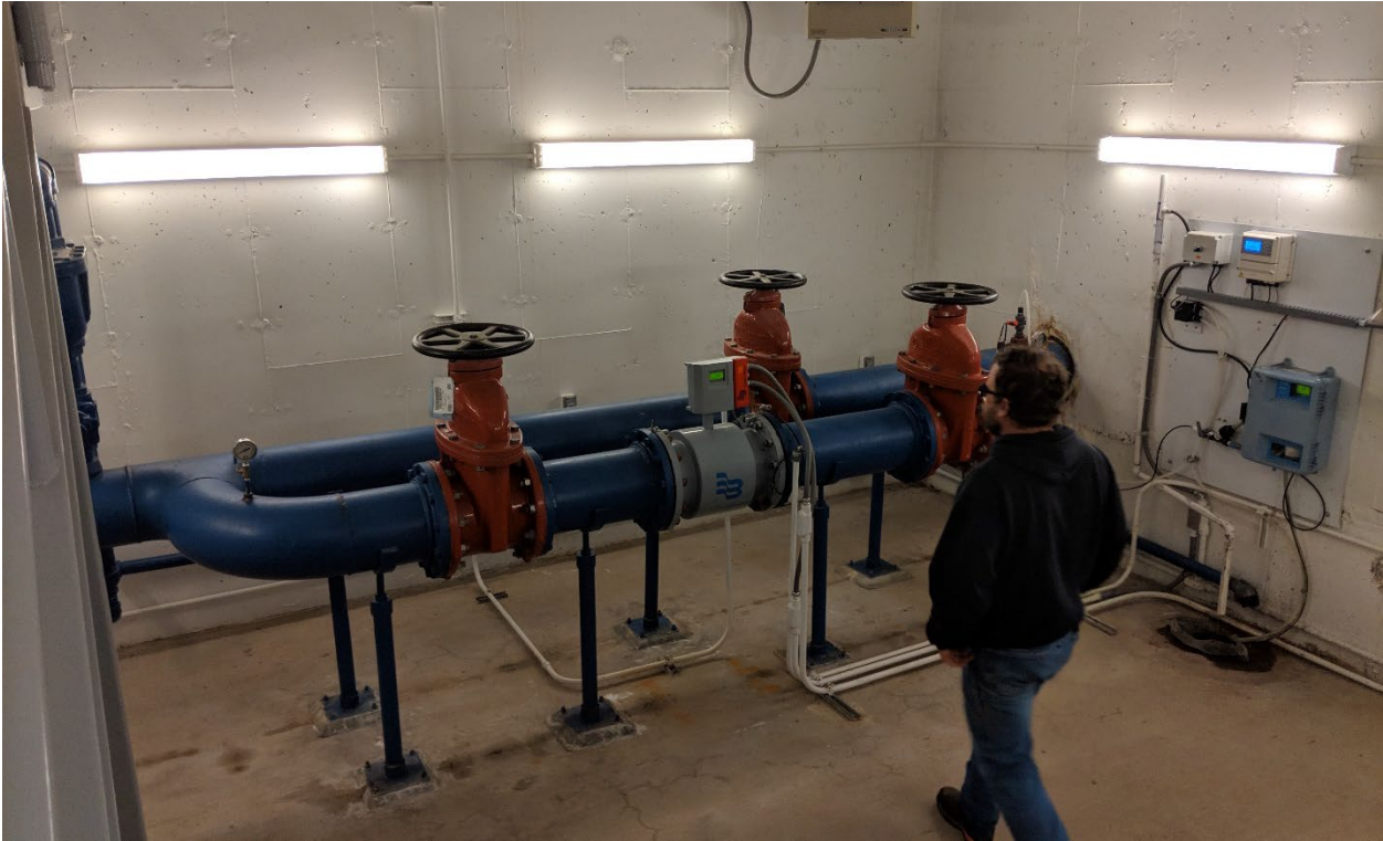
Figure 3.4: Chlorine Residual Building
