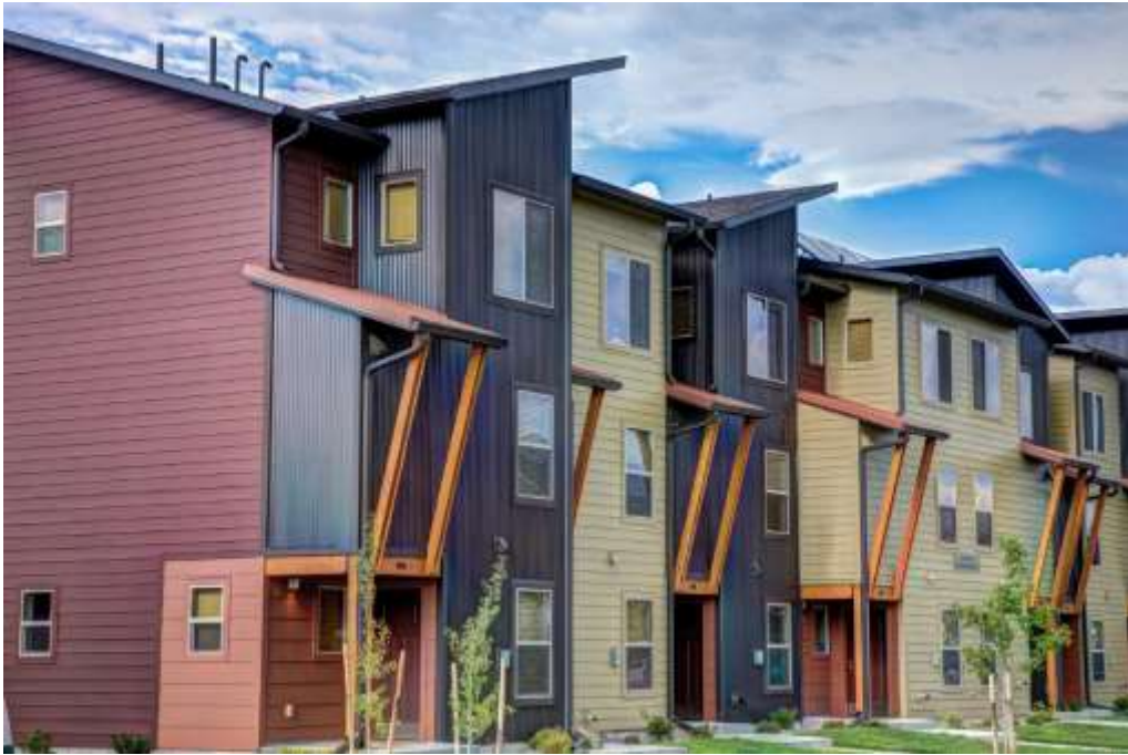
Figure 11. Three-story apartments and townhomes with parking to rear
