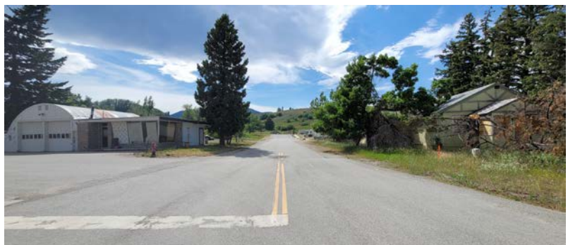
Figure 6. Abandoned buildings surround 2 nd street & Broadway. A lack of curb, gutter and sidewalks connect to the Mountain Springs Villa development
