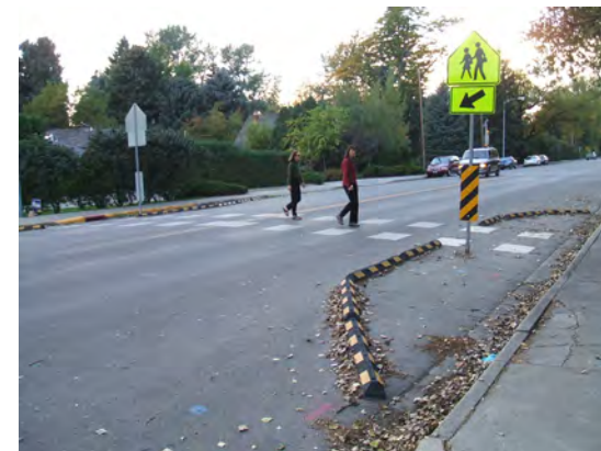
TEMPORARY PIN-DOWN CURB EXTENSION IMAGE COURTESY OF MARK FENTON
