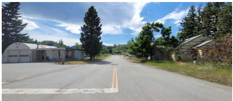
Figure 6. Abandoned buildings surround 2 nd street & Broadway. A lack of curb, gutter and sidewalks connect to the Mountain Springs Villa development
