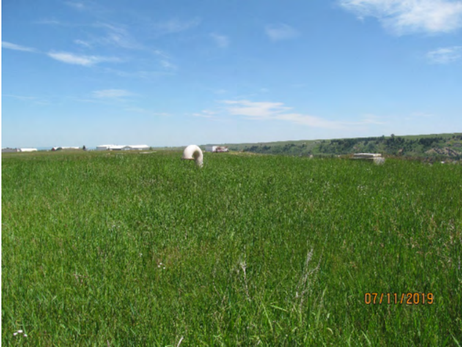
(ST001) Storage tank airport-single hatch and vent-750,000
