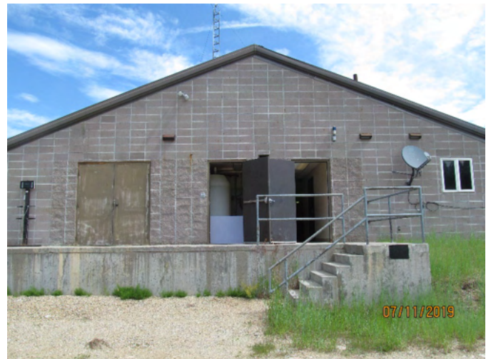
(TP003) exists inside surface water plant as water enters clearwell
