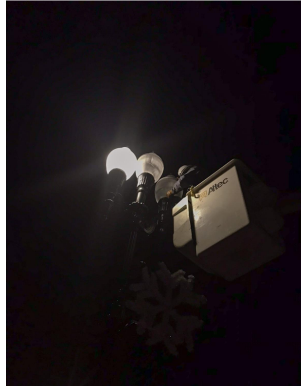
Above: Replacing City-owned bulb with a 3000k LED on the corner of 8th and Broadway
