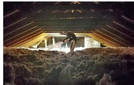
Insulation being installed at City Hall
