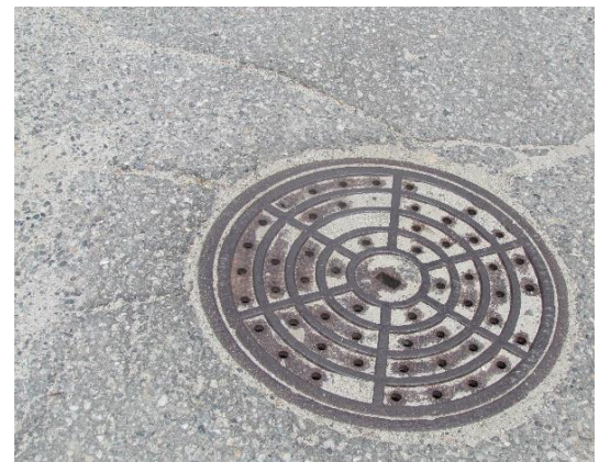
Manhole cover on Haggin Avenue
