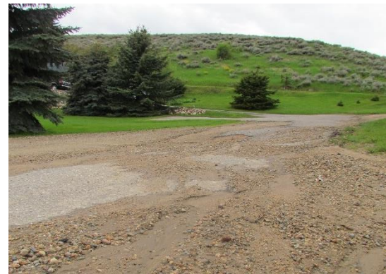
Stormwater runoff following a rainstorm in town
