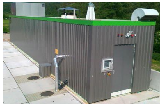
An example of an Anaerobic Digester
